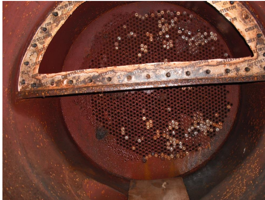
Figure 1 – A FWH with 28% tubes plugged
