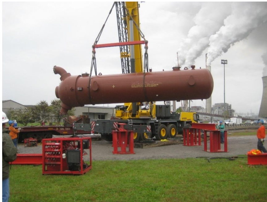
Figure 2 – Unloading a Replacement FWH
