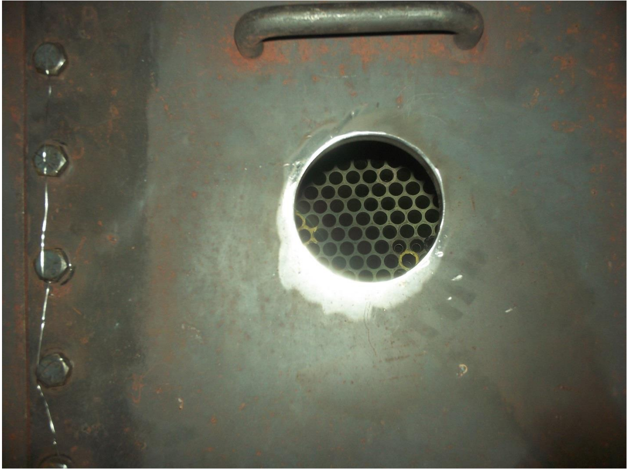
Figure 4 – Typical Orifice drilled in FWH pass partition plate
